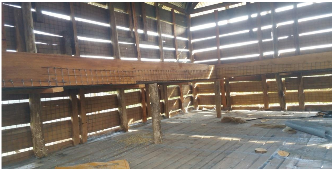
This shows how it was constructed inside. The raised part is for the beans then below it for maize.
